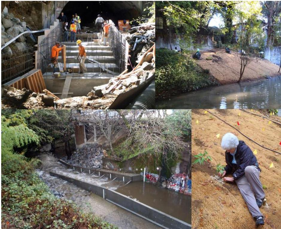
*Clockwise from top left: a Glissman Excavating crew installs forms for the fishway walls, as engineers check the work; giant reed was removed from a relatively steep slope, subsequently covered with erosion-control matting, into which a CCNB crew installs native plants; Sandy Goldman demonstrates that darned skills still have a place; the completed fishway, visible from Center Boulevard. Photos by Sandy Goldman and Charles Kennard*
