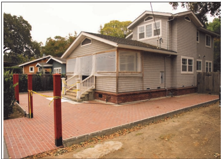
The paving over of the Ross Valley is the major cause of the decline of fish numbers in our creeks, because fast rainwater runoff alters winter and summer flows, and re-contours the stream channels. Photo by Charles Kennard
