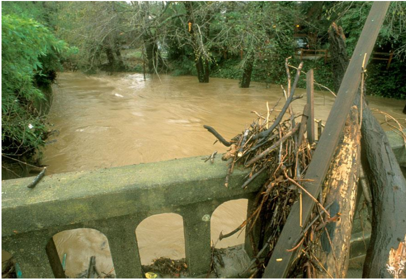
Nokomis Avenue bridge contributes to local flooding, and is due to be replaced. Photo by Charles Kennard
