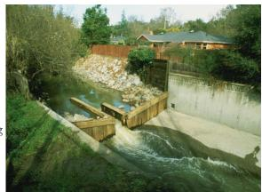
The fish ladder located at the upstream end of the concrete channel, broken and non-functional, also exacerbates water-level rise during flood events, when the flow breaches the channel along Sylvan Lane. Flood waters inundate Ross Common, and flow through buildings, streets, and gardens on their way to the Bay. Photo by Charles Kennard
