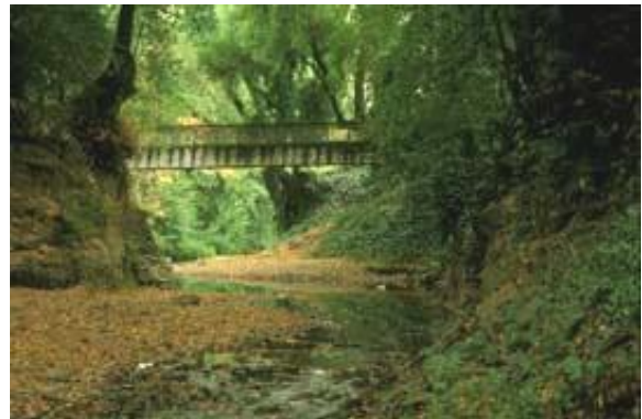
Sais Footbridge, spanning 75 feet, is made of laminated lumber, and lacks abutments that can catch debris during floods. Photo by Charles Kennard
