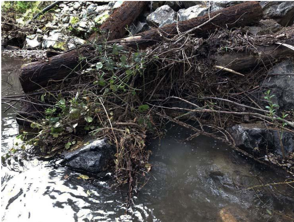
Structures such as this log, installed in Ross Creek, do triple duty: provide shelter for fish, protect the creek bank from erosion, and are convenient places to attach temperature gauges. Photo by Sandy Goldman
