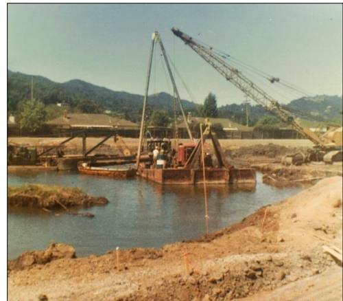
Before the concrete channel was constructed in Kentfield and Ross, the downstream reach was straightened and widened, and earthen berms constructed, as seen here near Bon Air Bridge in 1968. Photo courtesy of Richard Torney
