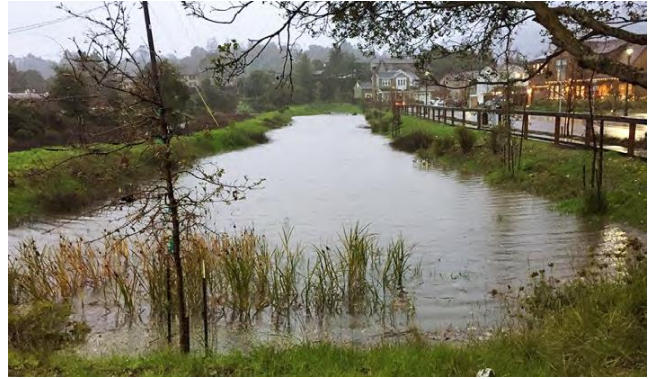
The swale, about 550 feet long, is located at the east end of the Rose Lane development, parallel to Larkspur Creek. The swale filled after a big December storm, and is seen from Doherty Drive. Photo by Sandy Goldman
