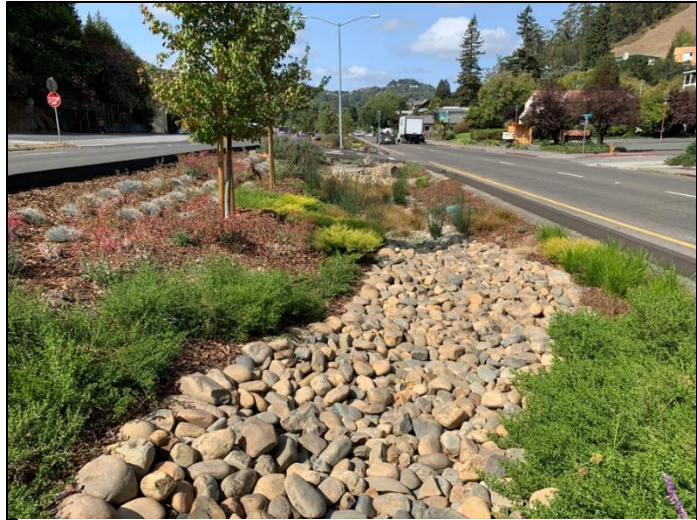
The median strip along San Anselmo's Miracle Mile was redesigned as a swale. Photo by Siegfried Engineering
