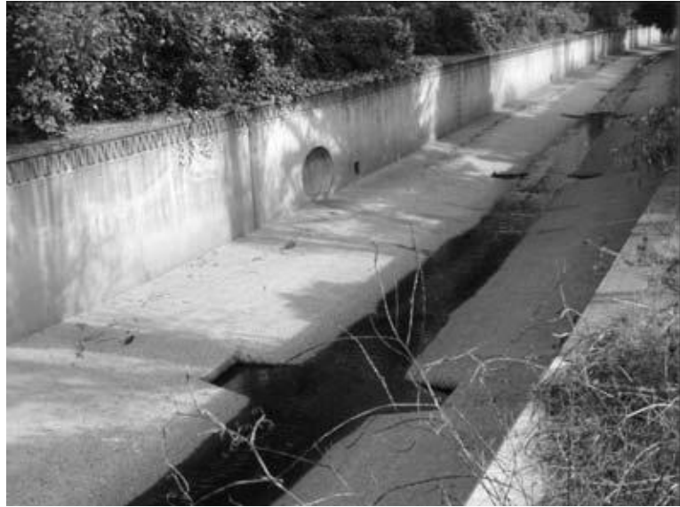
The concrete channel through Kentfield. Photo by Michael Love
