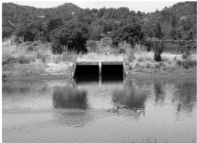
The mouth of the culverts conveying Tamalpais and Murphy creeks into Corte Madera Creek, downstream of the concrete channel in Kentfield. Photo by Sandy Guldman
