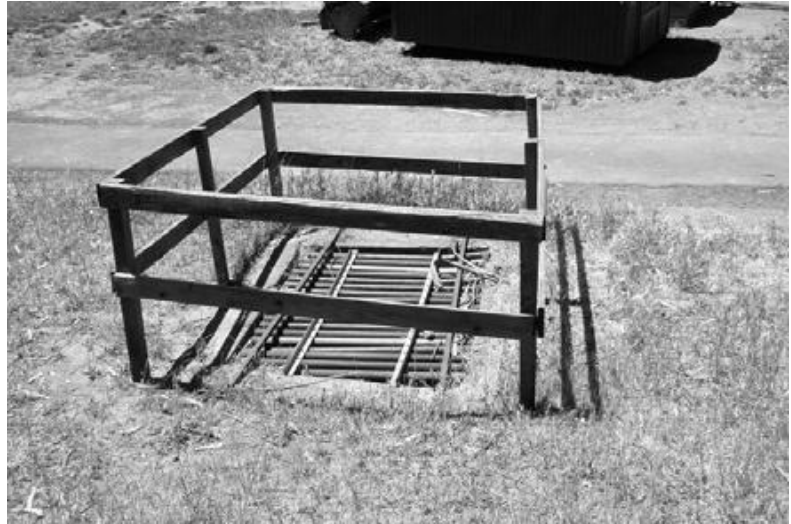
Sorich Creek culvert. Photo by Sandy Guldman
