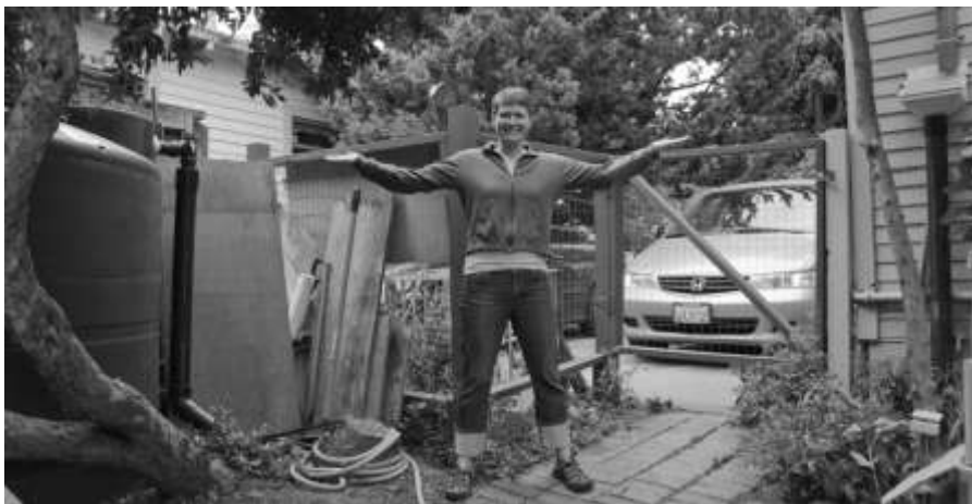
Pam Hartwell-Herrero, director of Sustainable Fairfax, stands between the standpipe (at the right edge of the picture) that receives inflow from the downspout and the 1,000-gallon tank that receives inflow via the pipe buried beneath the walkway. The system functions by gravity, with water drawn off by a hose bibb at the bottom of the tank. Photo by Sam Wilson
