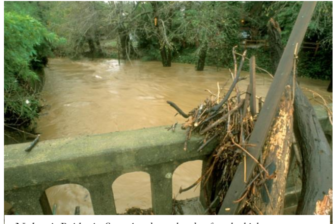
Nokomis Bridge in San Anselmo, shortly after the high water on 12/31/2005: It is one of several inadequate bridges that also cause flooding scheduled for replacement as part of the Ross Valley Watershed Program. Photo by Charles Kennard
