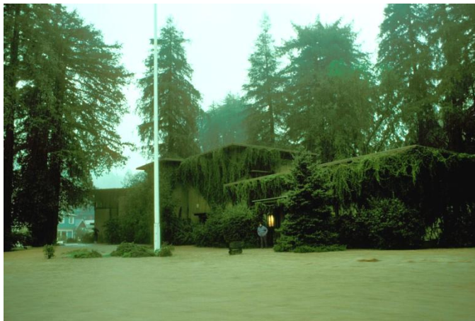
Flooding at Fairfax Town Hall in 1982: Installation of the Lefty Gomez and Loma Alta detention basins would lower flood waters in downtown Fairfax in flood events. Photo by Charles Kennard
