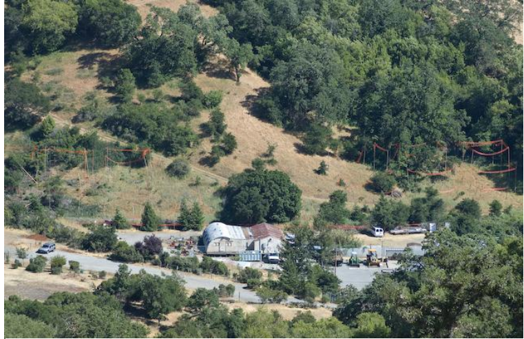
The eastern edge of the Sorich valley floor is dominated by San Anselmo's corporation yard. A tributary of Sorich Creek runs in a culvert on Town property, and also on adjacent private property, for which Jerry and Mea Draper have proposed a housing development. Story poles are visible in the photograph. Photo by Sam Wilson
