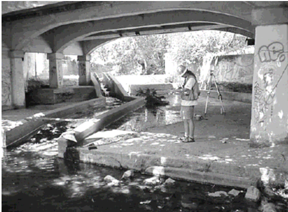
Preliminary Priority 1: Fish ladder with a long, narrow chute downstream, on San Anselmo Creek at Saunders Avenue (San Anselmo), Ross Taylor and Associates ©2003
