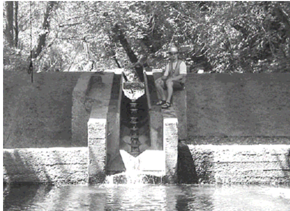
Preliminary Priority 2: Fish ladder on San Anselmo Creek at Pastori Avenue (Fairfax), Ross Taylor and Associates ©2003
