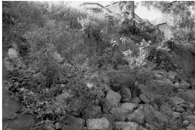
This San Anselmo site is subject to severe creek flows, but this biotechnical solution using riprap, cables, and native plants held firm during the New Year's Eve flood.
