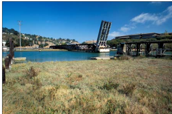
Corte Madera Creek at the railroad trestle, Larkspur
