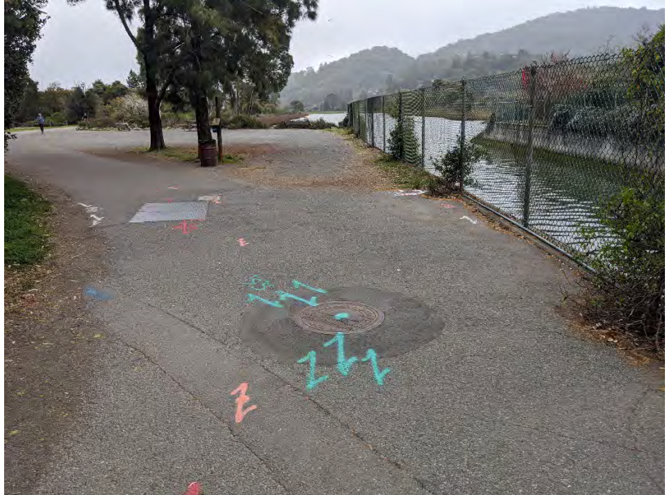
Photo 2. Looking downstream from the left bank paved multi-use pathway (MUP) where the sanitary sewer and other utilities running under the MUP turn approx. 45 degrees to the SE to depart from the edge of the channel and continue under or adjacent to the MUP. This photo also shows the flat triangular gravel-covered area with picnic tables and benches.
