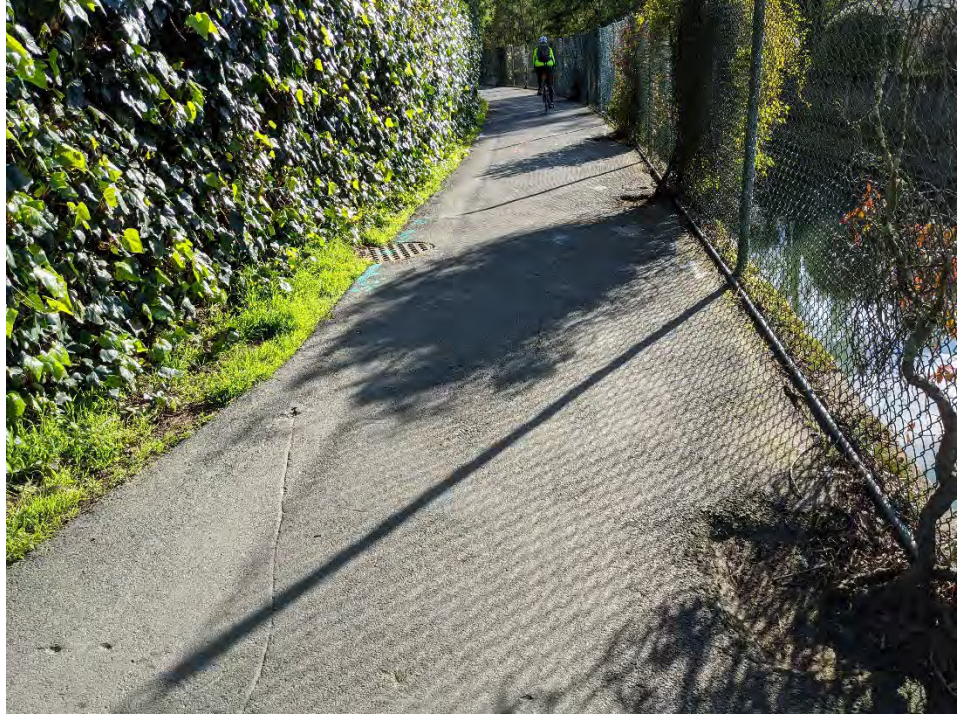
Photo 5. Looking downstream to the Multi-Use Pathway (MUP) running along the top of the left (east) concrete channel wall. Note the sanitary sewer (SS) manhole and green paint marking the SS utility line running under the pathway at depth and offset from the left channel wall.
