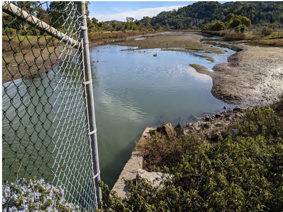
Photo 4. Looking downstream from the concrete channel terminus to the earthen channel beyond. Sedimentation in the earthen channel prevents tides lower than 1.7 feet NAVD88 from occurring in the project reach.
