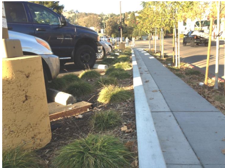
During a downpour, rainwater runoff from a parking area at Good Earth in Fairfax flows into planted areas rather than being directed into storm drains. Photo by Gerhard Epke
