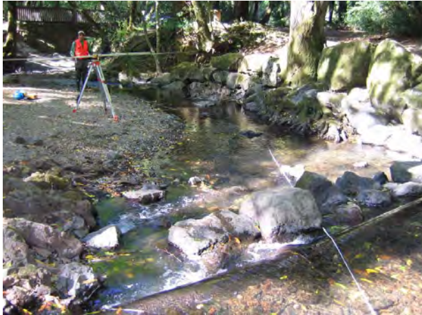
Figure 12: Water pipeline crossing Ross Creek
