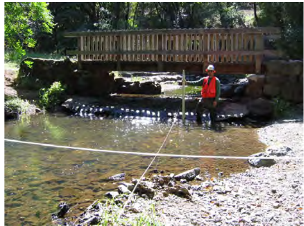
Figure 13: Pedestrian bridge with weir
