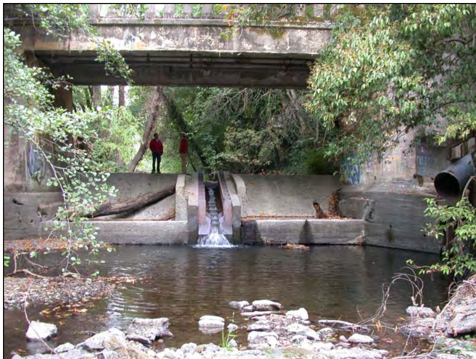
Figure 1 – The existing Pastori Ave. Bridge over San Anselmo Creek, with a concrete apron between the bridge abutments that functions as grade control. Poorly functioning Alaskan Steeppass fish ladder in center.
