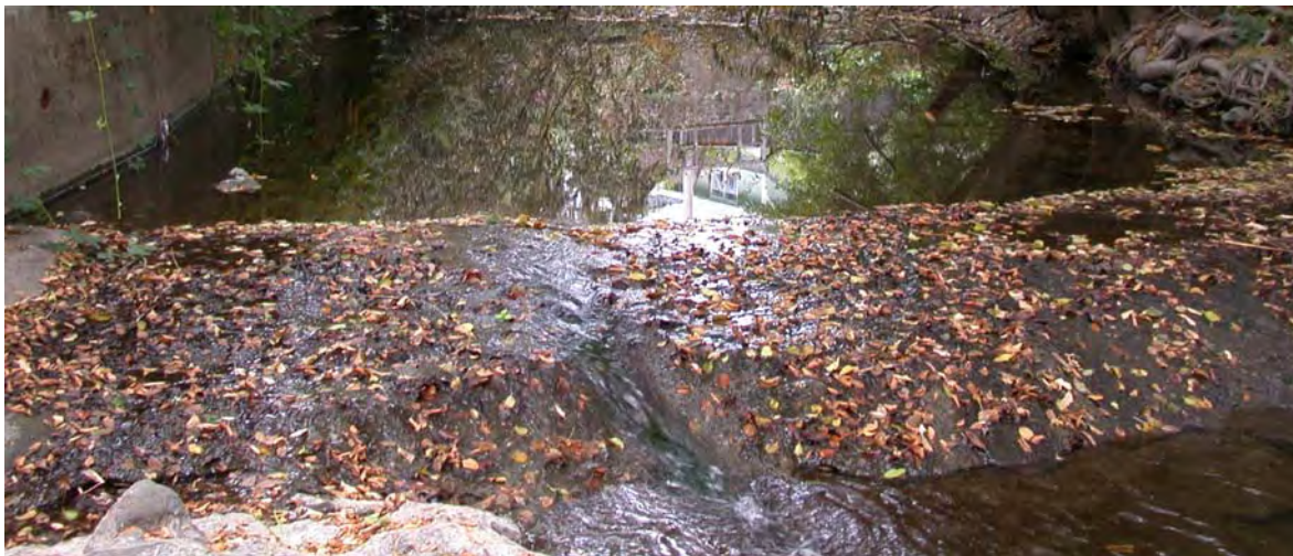
Figure 5 – Upstream sewer line encased in concrete. The fish ladder and bypass weirs are designed to backwater the exposed concrete to facilitate juvenile passage at low flows.
