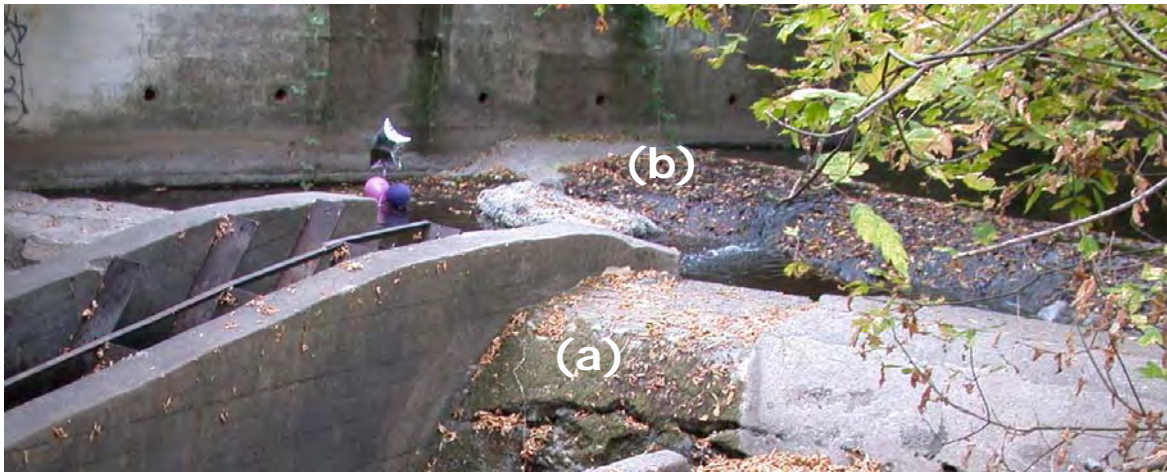
Figure 2 – Looking upstream at existing fish ladder exit. Two sewer pipes cross the channel encased in concrete (a) at the weir across the apron, and (b) approximately 12 feet upstream of the apron.
