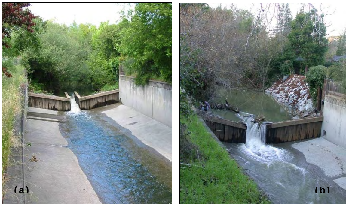
Figure 1 – Existing Denil fish ladder and bypass weirs at the upstream end of Unit 3 (a) during low-flow in June 2005 and (b) in January 2006, following the New Years flood.
