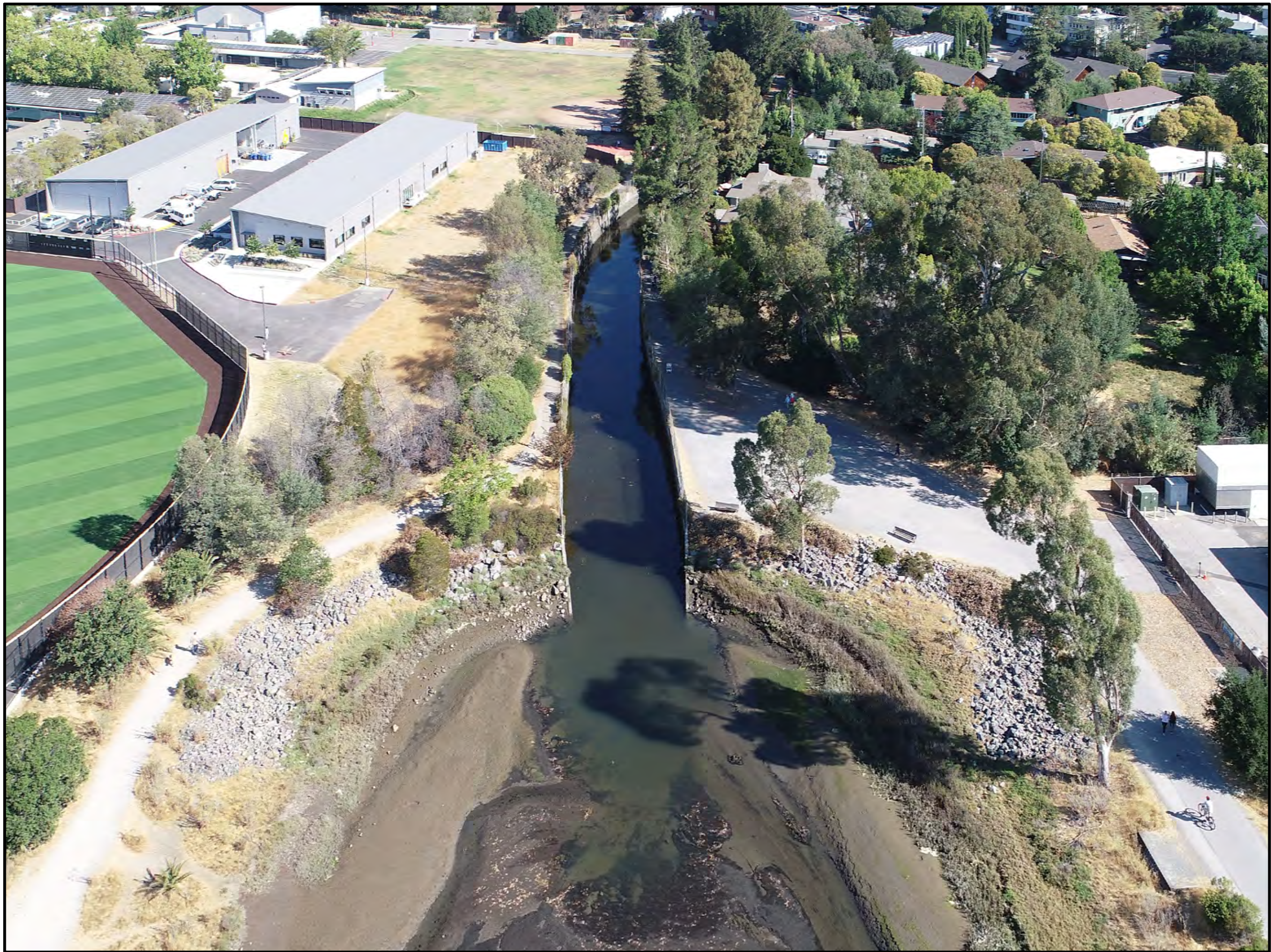
EXISTING CONDITIONS DATE OF FLIGHT: 10 AUG 2021 (~1.8' NAVD88) (SEDIMENTATION IN THE EARTHEN CHANNEL DOWNSTREAM FROM THE CONCRETE CHANNEL PREVENTS TIDE LEVEL IN THE CONCRETE CHANNEL FROM REDUCING BELOW RIFFLE ELEVATION (APPROX. 1.7' NAVD88, NOT SURVEYED).
