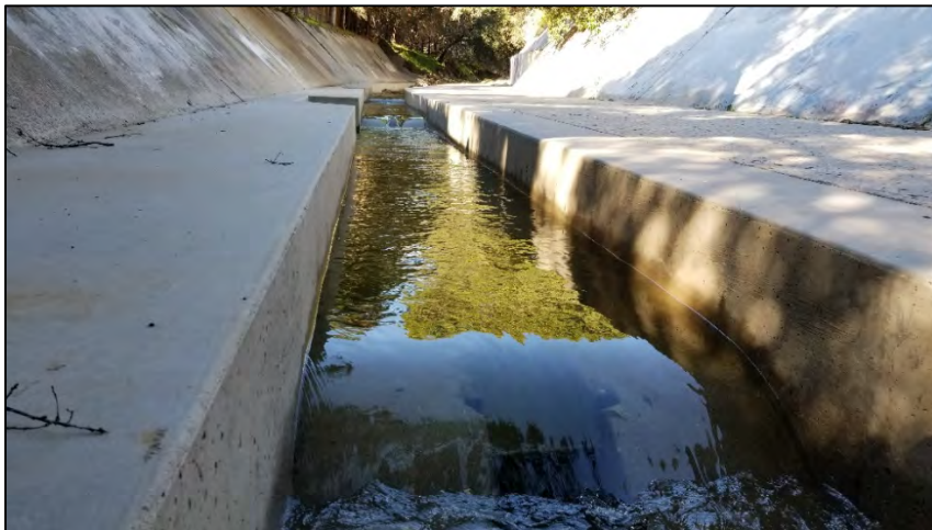
Figure 2. Mission Creek fish passage retrofit with low-flow channel, pocket pools, and rounded weirs to control depth (bottom photo: M. Garelo).
