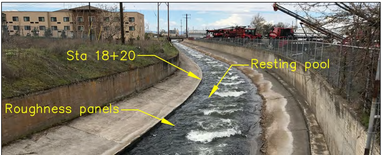
Figure 3. Mill Creek flood control channel fish passage modifications, replacing a baffled low-flow channel (top left) with new baffles, roughness panels, and resting pools (top right and bottom) (photos from TriState Steelheaders and Patrick Powers).
