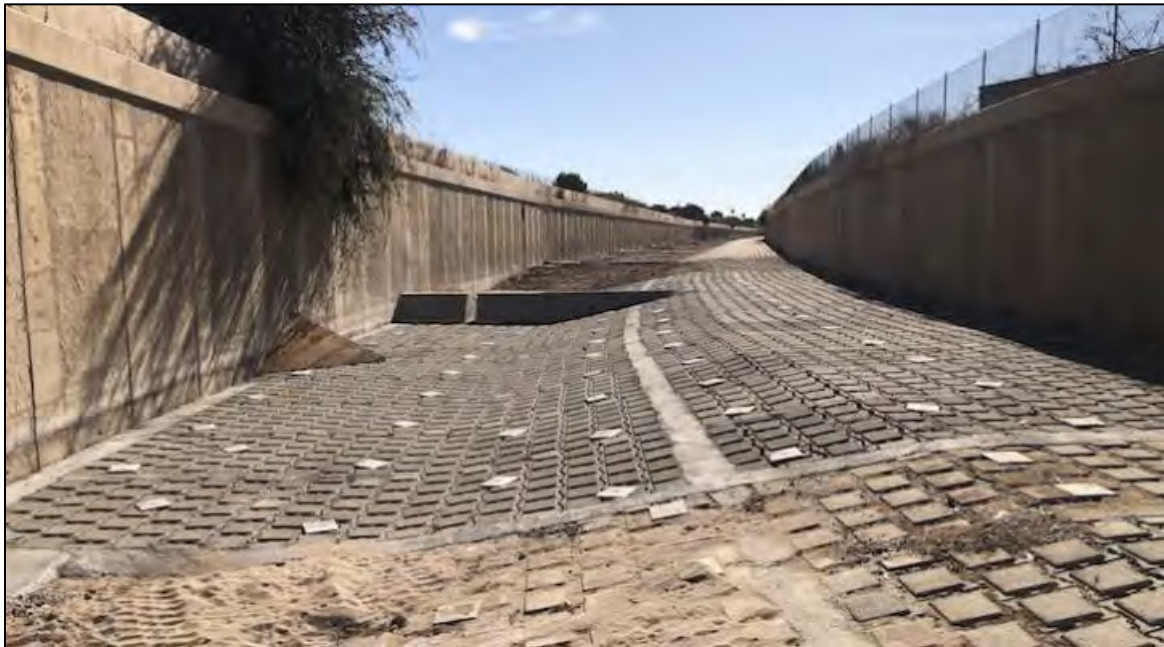
Figure 4. San Jose Creek flood control channel with rounded baffles for passage of adult Steelhead (top photos: Ed Zapel; bottom photo: City of Goleta).
