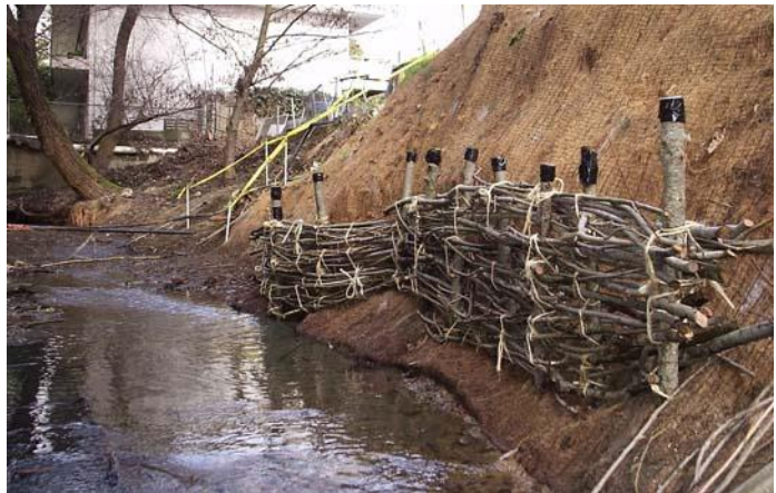
In this special application, a woven willow fence with living stakes was used to protect a slope from erosion by high waters. Photo by Vicki Burns
